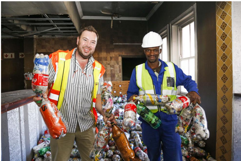
GVK's Johan Bosch and Fuzile Ntsume who managed quality control at a site level
